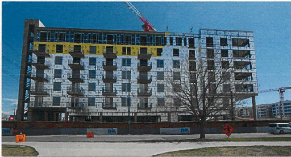
Greenhaus Under Construction in Sun Valley
