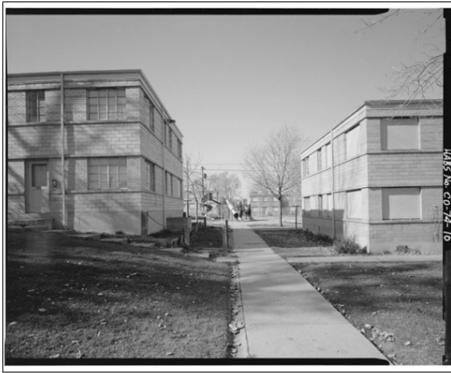
Image 10: The Historic American Building Survey (HABS) documented the Lincoln Park Homes project before it was demolished in 1994. HABS is a program of the National Park Service that documents buildings and places important to American history. Lincoln Park Homes was documented because it was one of Colorado's earliest housing projects. Photo c.1990. Credit: Library of Congress, Prints & Photographs Division, HABS, CO-74.
