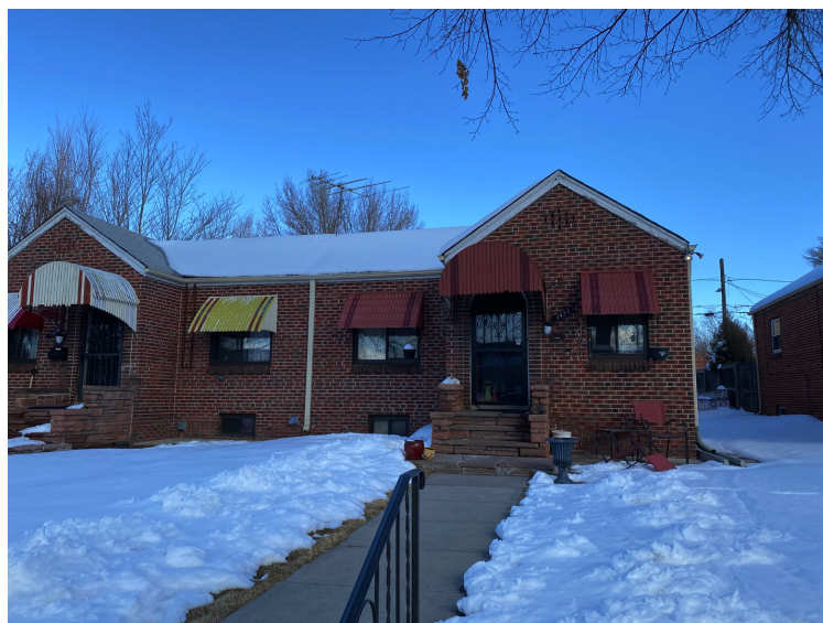
Image 12: Over the decades, DHA has acquired and rehabilitated many single- and multi-family homes to improve the overall quality of life in Denver's neighborhoods, such as this duplex in the Hale neighborhood. Photo c.2021. Credit: Denver Housing Authority.
