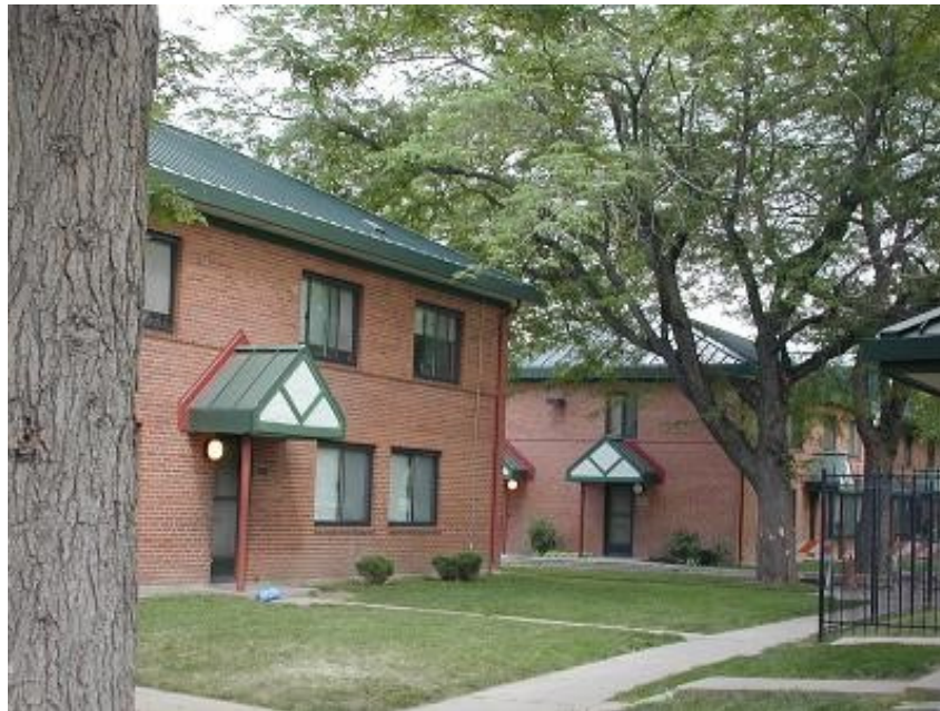
Image 3: Platte Valley Homes was completed in the Five Points Neighborhood by DHA in 1942. The project was funded by the U.S. Housing Authority, and the simple, unornamented two-story brick buildings were typical of affordable housing from the 1940s. Year of photo: unknown. Credit: Files of the Denver Housing Authority.
