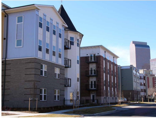
Image 9: Block 1 of the Curtis Park HOPE VI development. Completed in 2007. Photo: 2008. Credit: DenverInfill Blog, Ken Schroeppel.
