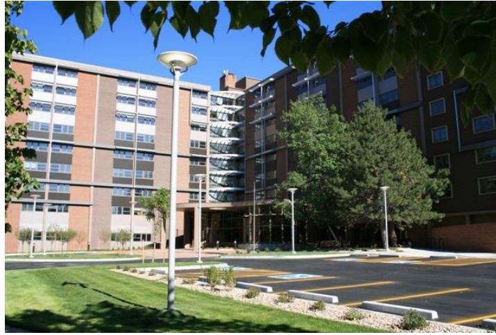
Image 6: Hirschfield Tower is a nine-story residential tower that opened in 1967 for seniors. It exhibits many characteristics typical of mid-twentieth-century residential towers that followed the design tenets of the Modern movement. The layout of the tower was specifically designed to meet the special needs of seniors. Date: unknown. Credit: Denver Housing Authority.
