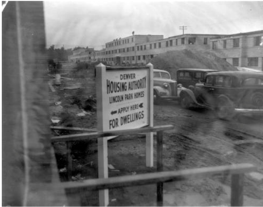
Image 5: Construction of Lincoln Park Homes (bounded by West Colfax and 13th Avenues and Mariposa and Osage Streets) in c.1940. A sign reads, "Denver Housing Authority: Lincoln Park Homes, Apply Here for Dwellings.". Credit: Denver Public Library Special Collections [call number X-29034].
