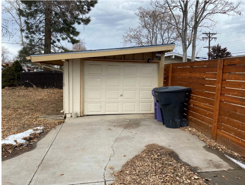
Image 26: By the time the Cliff May homes in Harvey Park were built in the mid-1950s, American families relied on personal vehicles for transportation, so garages were incorporated into many properties. Photo c.2021. Credit: Denver Housing Authority.
