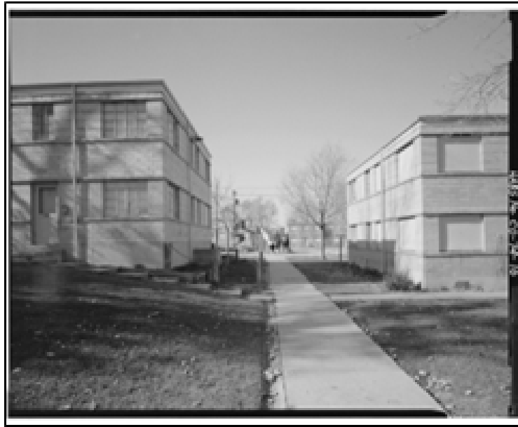
Image 14: The Historic American Building Survey (HABS) documented the Lincoln Park Homes complex (at the corner of West Colfax Avenue and Mariposa Street) before it was demolished in 1994. HABS is a program of the National Park Service that documents buildings and places important to American history. Lincoln Park Homes was documented because it was one of Colorado's earliest housing projects. Photo c.1990. Credit: Library of Congress, Prints & Photographs Division, HABS, CO-74.
