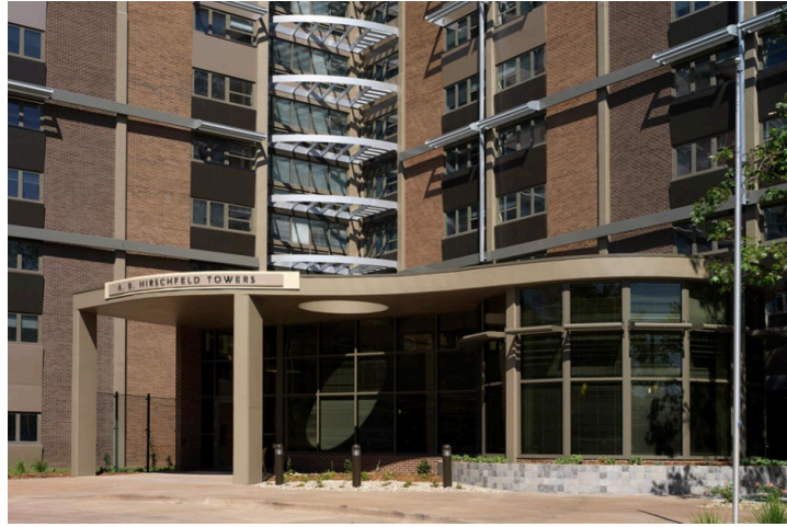
Image 36: Piano-shaped lobby that serves as the main entrance into Hirschfeld Towers. Photo c.2009. Credit: Santulan Architecture.
