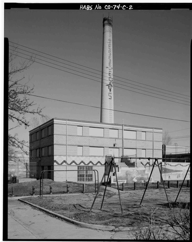
Image 16: A c. 1990 photo of Lincoln Park Homes, including one of the residential buildings with part of the on-site power plant in the background and a playground in the foreground. Credit: Library of Congress, Prints & Photographs Division, HABS, CO-74.
