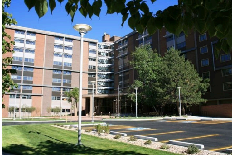
Image 33: Southeast side of Hirschfeld Towers. Credit: Denver Housing Authority.
